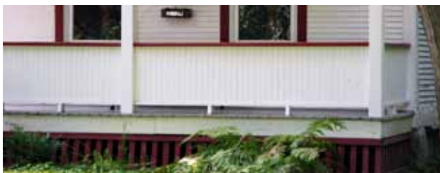
Garde-corps plein, Saint-Pie
